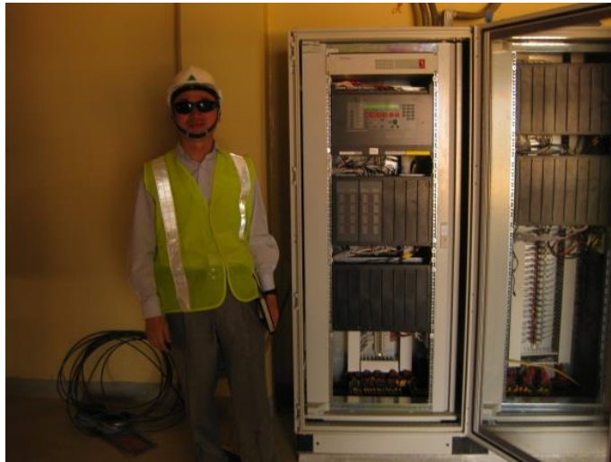
DTS (top) rack-mounted solution
